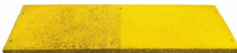
Example showing before and after high pressure cleaning
